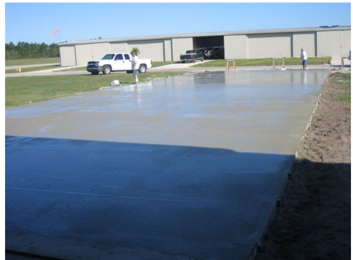
Installation of the new hangar ramp
