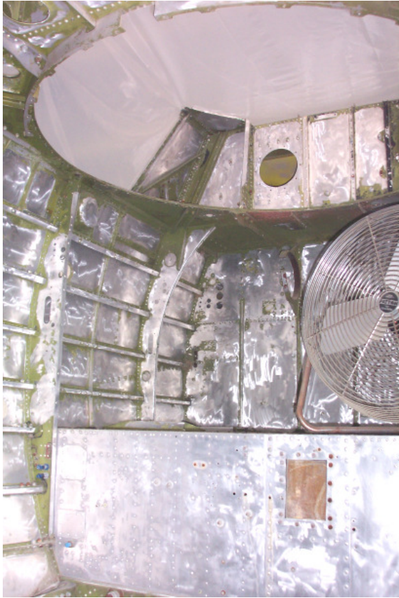
Interior bead blasting
